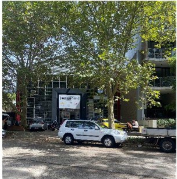
View looking west on Young Street along frontage of site.
